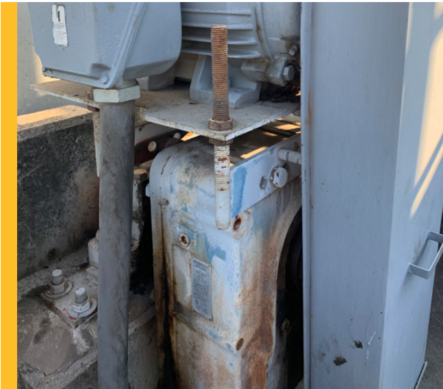
The existing belt-driven system with an obsolete gear reducer was inefficient and laborious to maintain, requiring frequent inspections by two technicians.
