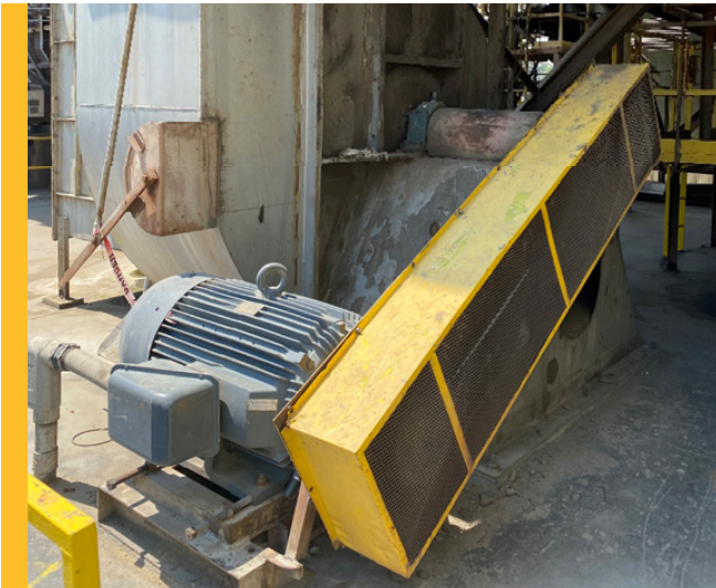
The circulation of hot air through the chamber is controlled by large forced-draft fans, crucial to production and utilizing 4-15/16 inch SAF-style bearings.
