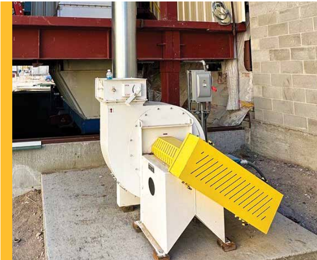
Imperial ISAF bearings are being installed on all air relief system fans in the manufacturing facility due to reduced maintenance and superior performance.
